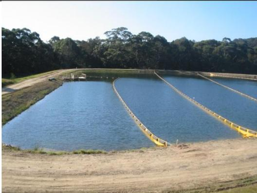
HDP-Baffle-3m in waste water treatment plant detention pond
