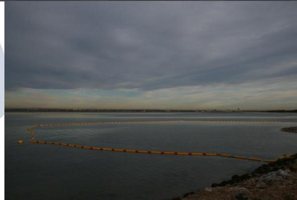
HDP-Silt-3m skirt deployed around dredge launching ramp contoured shore ends
