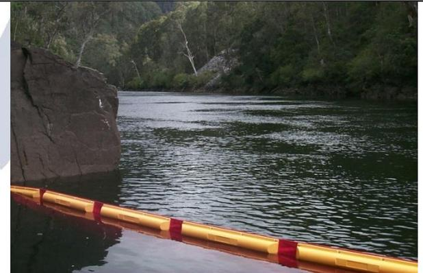
HDP-Debris-1m used as a tail race boom Tumut 1 power station. Subject to sub zero conditions
