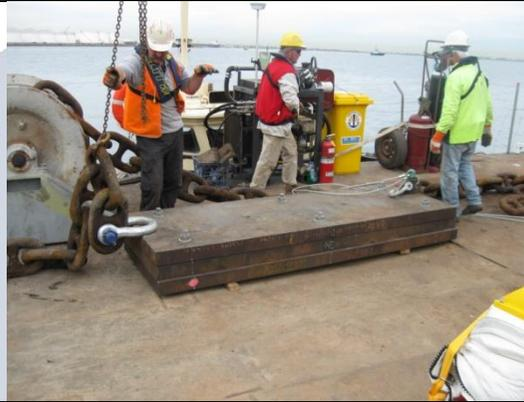
Typical end mooring steel dump ballast mooring, mooring chain 90-100mm stud link
