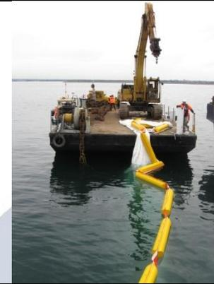
Sea-Curtain-Silt-10m being deployed from barge, ballast mooring concurrently deployed
