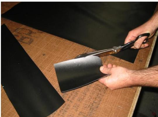
Cut appropriate patch from patch material provided ensuring corners on patch are rounded.
