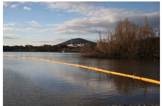
Curtain with skirt dropped and anchored
