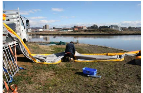
Curtain sections being joined
