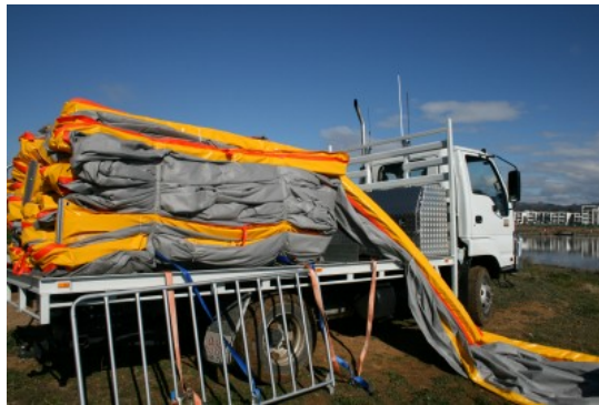
Furled curtain deployed from truck
