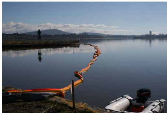
Furled curtain deployed into water
