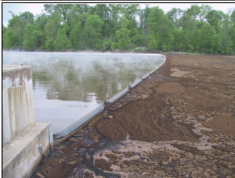
Figure 3: Floating baffle fitted with filtering flow through windows to limit sludge movement in pond
