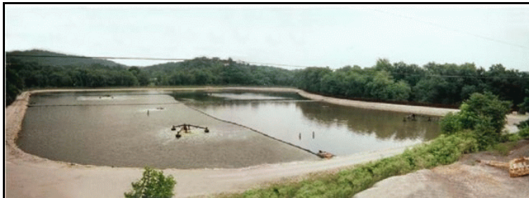
Figure 1: Typical floating baffle installation dividing a waste water pond into four treatment cells. Flow is controlled between each cell through the use of flow through windows.
